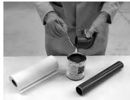
Applying the cement
