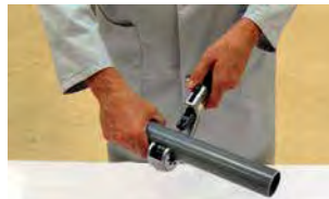
Cutting the pipe to length
