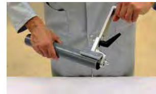
Chamfering the pipe
